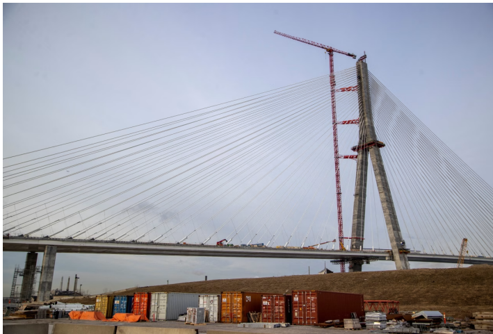
The Gordie Howe International Bridge under construction in Windsor, Ontario. CARLOS OSORIO/REUTERS
